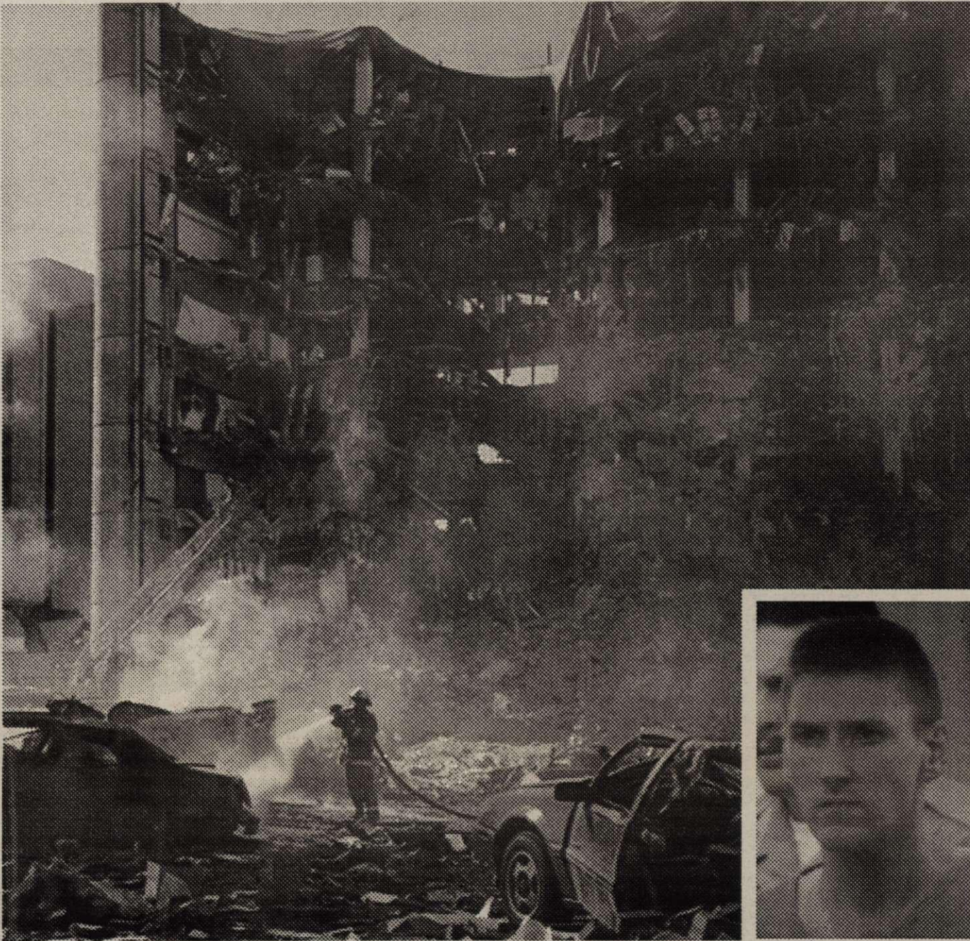
The Murrah Building in Oklahoma suffered tremendous damage from a car bomb.
