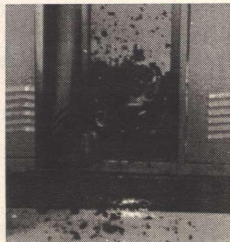
Ashes and burnt debris illustrate the extent of the fire.
