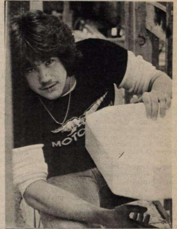
Carmine Capparelli repairing a sink.
