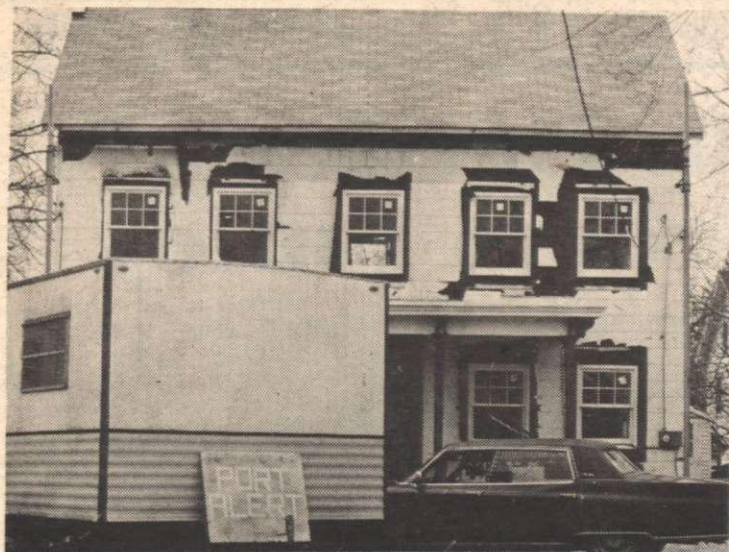
Port Alert building under reconstruction.
